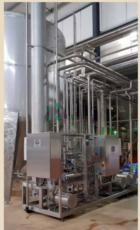
Fig. 1 Column water deaeration unit
